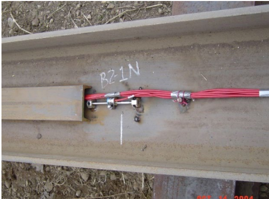
Figure 29. External surface-mounted VW strain gauges mounted on H-pile web.
