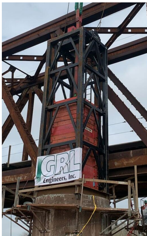
Figure 6. APPLE VIII with 80-ton ram testing a 10 ft diameter drilled shaft.
