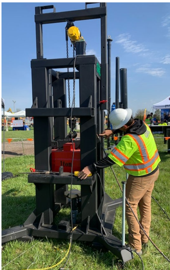
Figure 5. APPLE VII 2G with 1-ton ram testing a helical pile.
