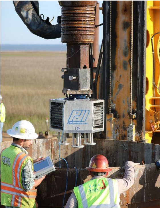
Figure 43. SQUID moving over shaft excavation.
