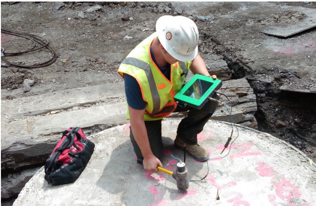
Figure 25. Low strain pile integrity test
