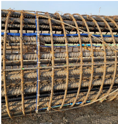
Figure 30. Sister-bar strain gauges attached to drilled shaft cage prior to embedment.
