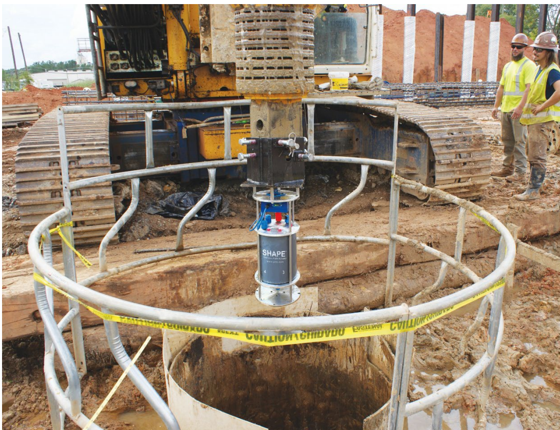
Figure 40. SHAPE moving over shaft excavation.
