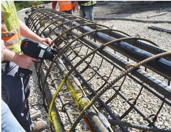
Figure 13. TIP wire attachment to a drilled shaft cage.
