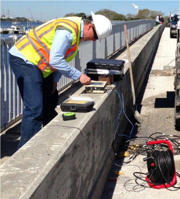
Figure 51. Parallel seismic test equipment.
