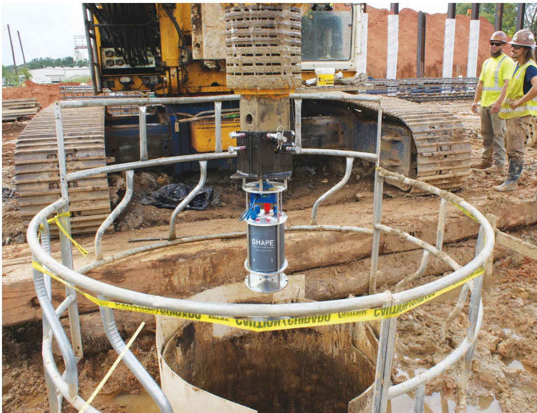
Figure 40. SHAPE moving over shaft excavation.
