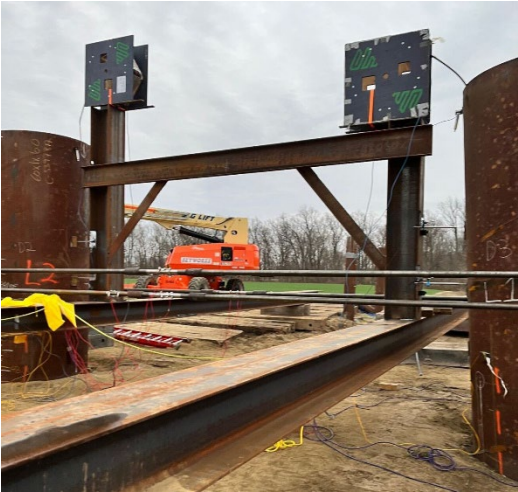
Figure 32. ShapeArrays installed in two pipe piles during a lateral load test.
