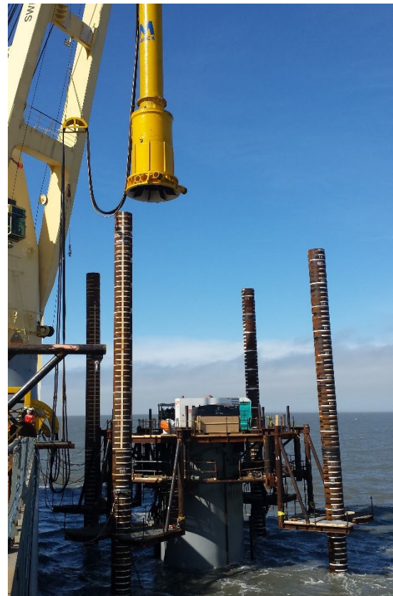
Figure 50. Platform with Underwater Testing.
