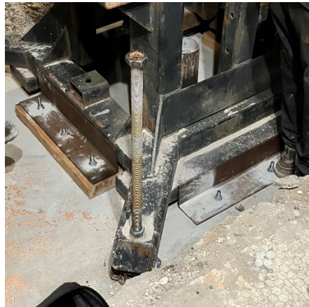
Figure 8. Anchoring system utilized to provide stability to dynamic load testing frame.
