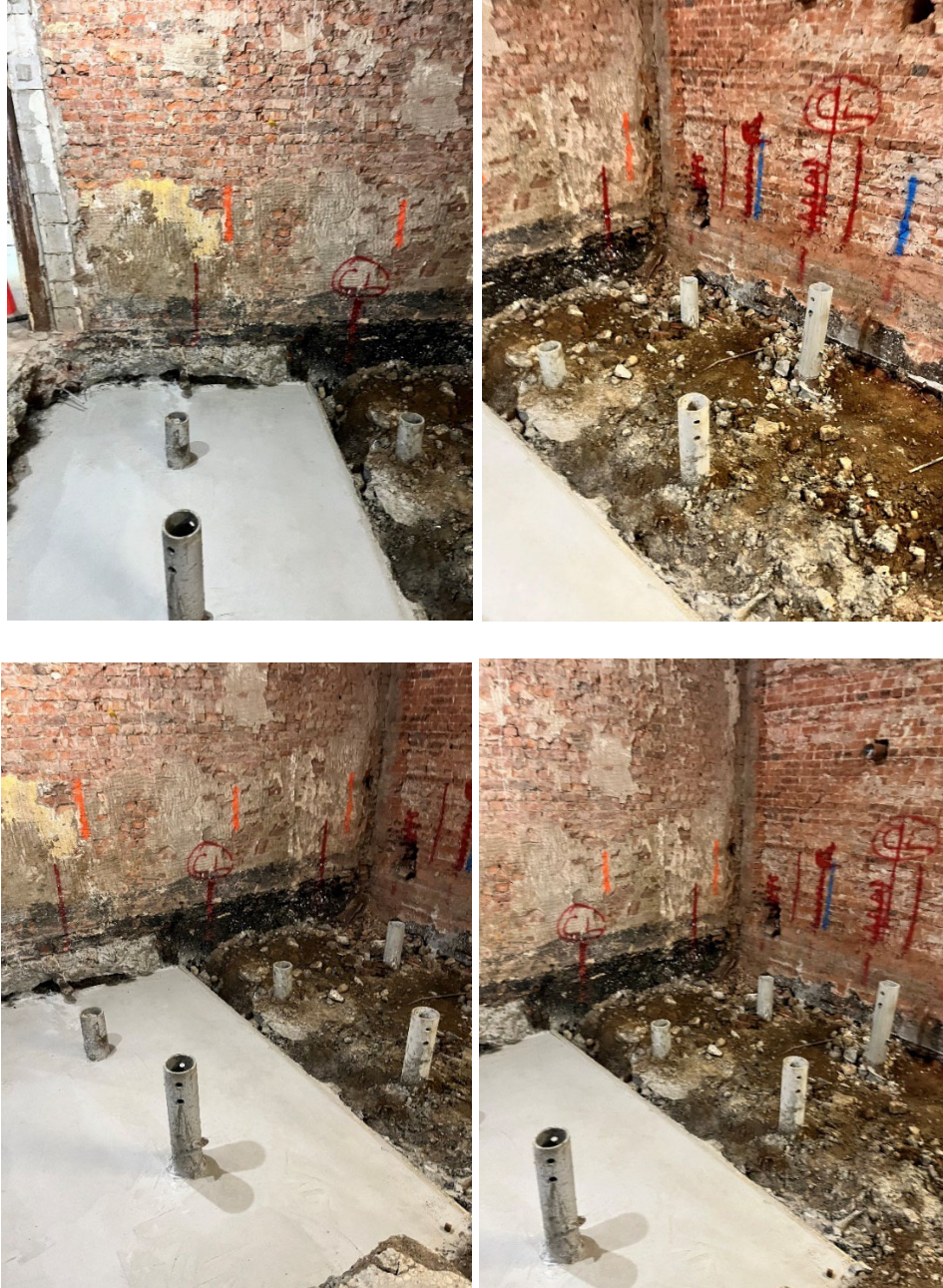
Figure 5. In-place conditions of the DDM inside the elevator shaft.
