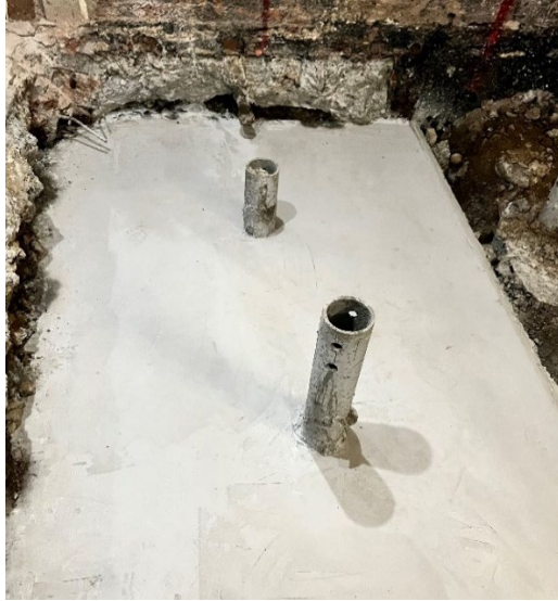
Figure 7. Poured concrete pad for dynamic load testing frame stability.
